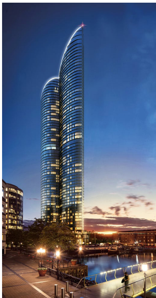
Tallest residential tower under construction in Canary Wharf. Photograph by Getty Images
