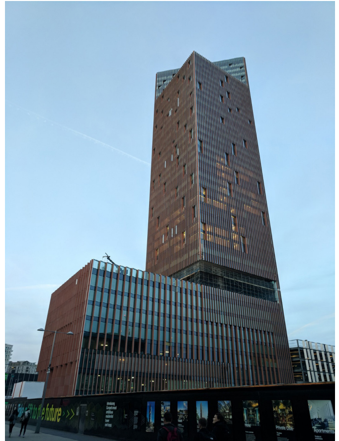
Manhattan Loft Gardens Photograph by The Wup
