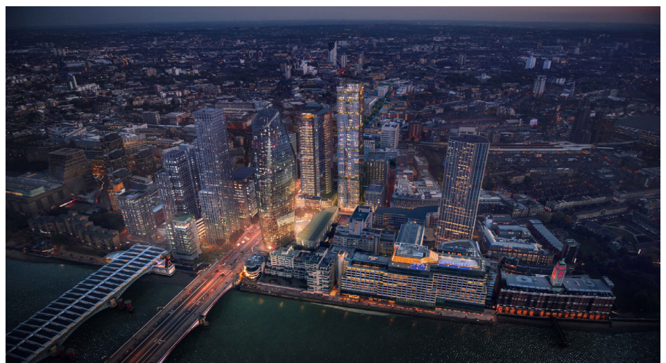
Southwark developments underconstruction Photograph by Getty Images
